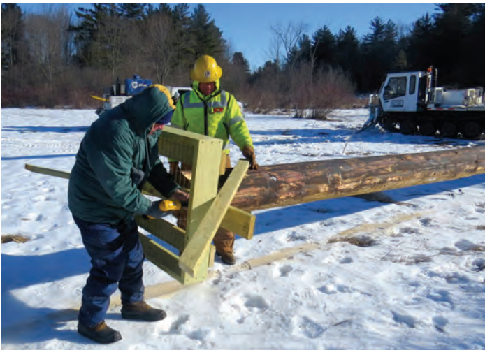
The new platform is attached to the new pole. Photo by Sue Bickford, Dover, NH, 2-26-19.
